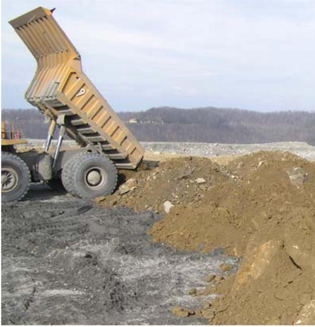
**Photo 1.** Loose dumping a topsoil substitute over a compacted subsurface on a West Virginia surface mine. The topsoil substitute material is being dumped in closely spaced piles and will be graded using only a single dozer pass. The final surface will be revegetated with a tree-compatible groundcover and trees will be planted in the loose topsoil substitute materials.
